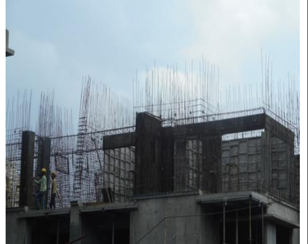
Project site-Naikenaware Buildcon Pvt Ltd-Neelaya, Talegaon(RCC structure upto parking then Mivan construction above parking )
