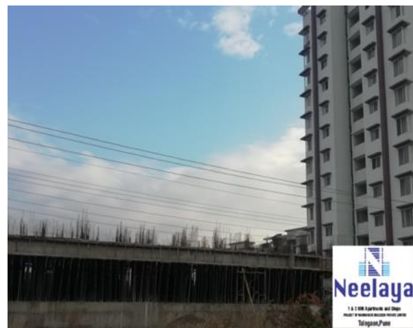
Project site-Naikenaware Buildcon Pvt Ltd-Neelaya, Talegaon(RCC structure upto parking then Mivan construction above parking )
