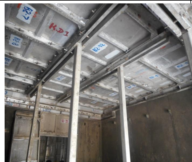
Slab and stair case in Aluminium formwork, M30 grade high strength concrete used for construction
