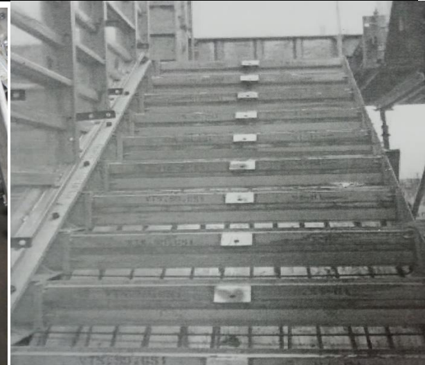
Slab and stair case in Aluminium formwork, M30 grade high strength concrete used for construction
