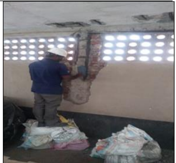
Site Visit of M.E. Civil students at "Jolly Maker Tower-1" at Nariman Point Mumbai showing repairing work for the column affected by Salinity and humidity by coating reinforcement and applying polymer modified mortar on 28 th November 2019
