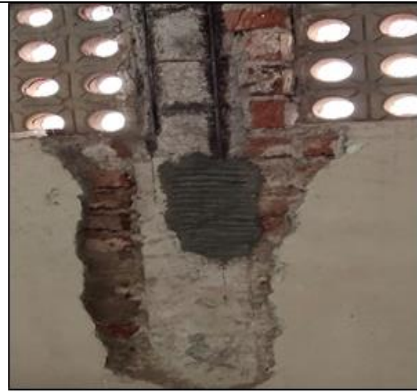
Site Visit of M.E. Civil students at "Jolly Maker Tower-1" at Nariman Point Mumbai showing repairing work for the column affected by Salinity and humidity by coating reinforcement and applying polymer modified mortar on 28 th November 2019
